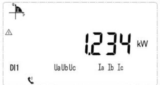
Current total power is 1.234kW
