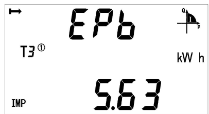
Current forward active energy on B phase
